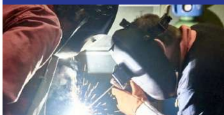
SUPERVISION ET CONTROLE QUALITE
